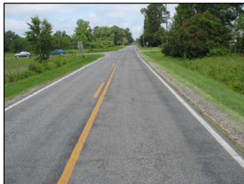
Figure 2: Westbound approach to the intersection.
