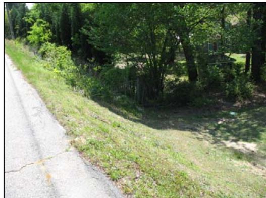
Figure 2: Steep slope of the grass-surfaced embankment.
