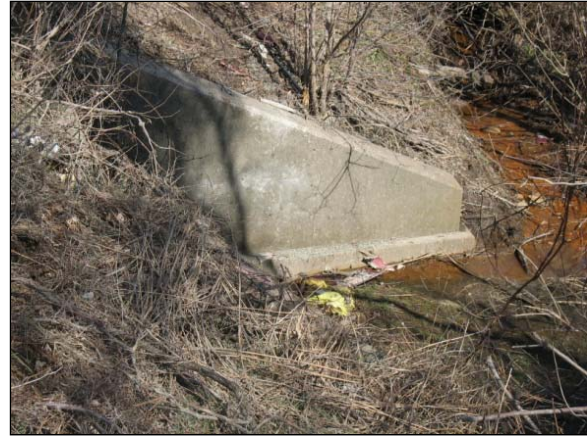
Figure 8: View of the concrete culvert wall impacted by the top plane of the Saturn.
