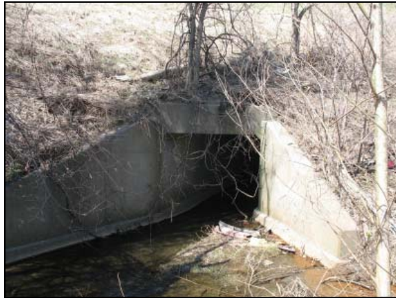
Figure 6: Northward view of the culvert and its headwalls.
