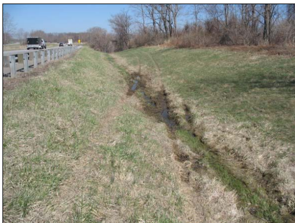
Figure 4: Off-road trajectory of the Saturn crossing through the swale and along the embankment.
