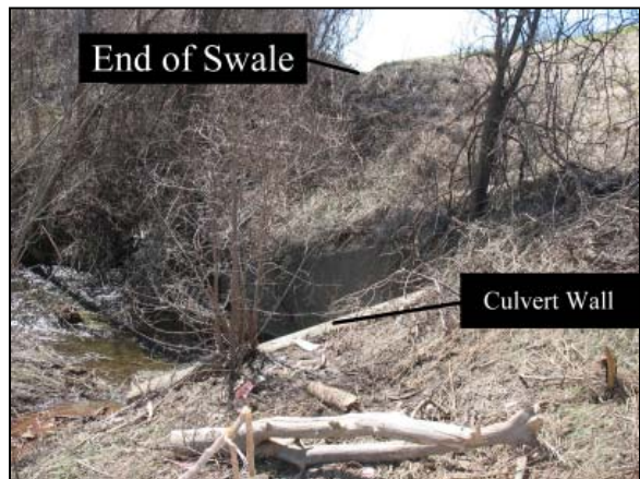
Figure 5: Look back view from the base of the ravine toward the end of the swale and the Saturn's trajectory.
