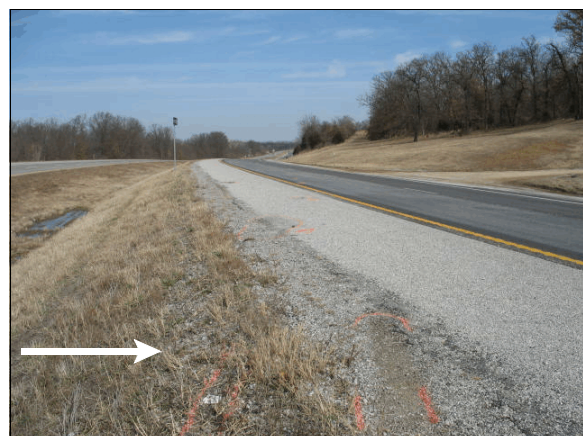
Figure 4: Arrow shows area where vehicle tripped and began to rollover driver side leading
