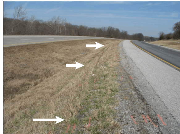
Figure 3: Orange paint marks and arrows show Honda's path of travel along the embankment
