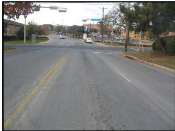
Figure 5: Westbound trajectory view 30 m (100 ft) from the intersection.
