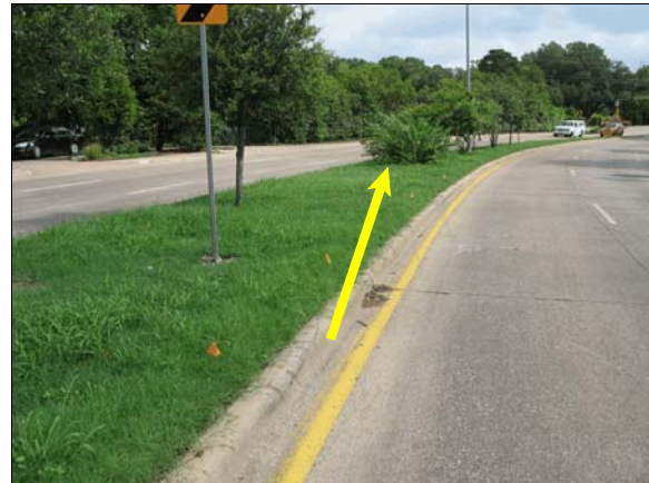
Figure 3: Chevrolet's median curb and shrub impacts (arrow shows path of vehicle)
