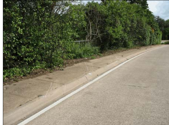
Figure 7: Area of multiple impacts on northwest side of south travel lanes
