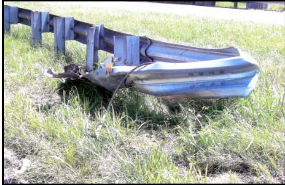
Figure 3: View of the damaged guardrail.
