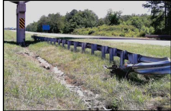
Figure 4: South view at the crash site depicting the guardrail impact and roll trajectory. The Mazda came to rest at the base of the pillar.
