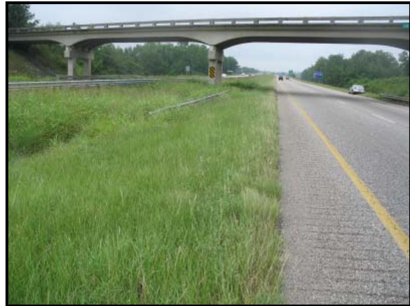
Figure 2: Southbound trajectory view in the area of the roadside departure.
