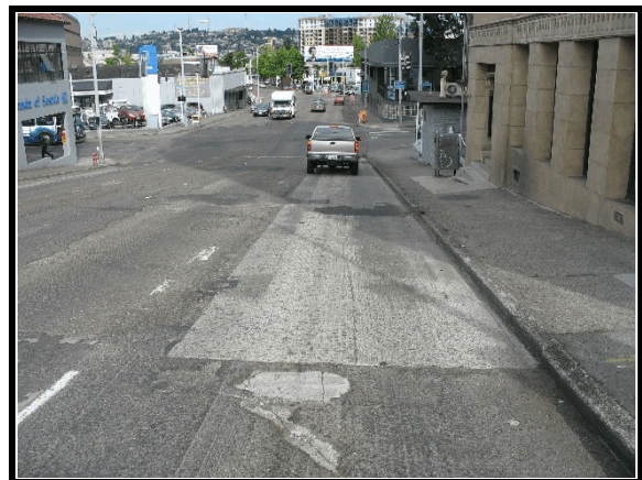
Figure 2. North approach for the 2008 Smart Fortwo
