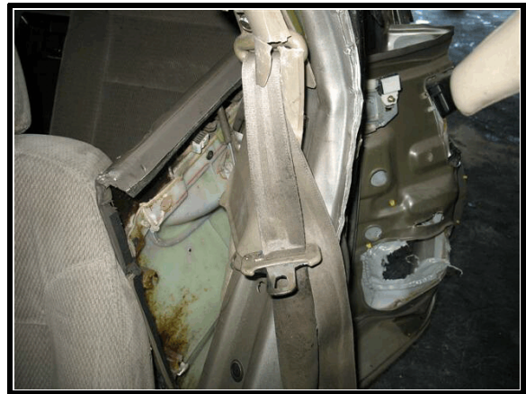
Figure 8. Driver's safety belt showing fracture of B-pillar cover
