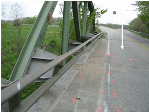
Figure 5: The back of Pontiac impacted the west bridge rail; arrow shows area of impact between front of the Chevrolet and left side of the Pontiac
