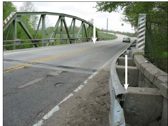
Figure 4: Arrow on right shows location of Pontiac's impact with end of east bridge rail and concrete bridge rail anchor, arrow on left shows area of impact with the Chevrolet
