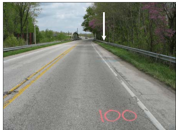
Figure 3: Northbound approach of Pontiac; arrow shows area of Pontiac's initial guardrail impact (guardrail had been replaced)
