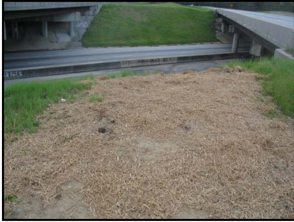
Figure 4: Post-impact trajectory view at the embankment.
