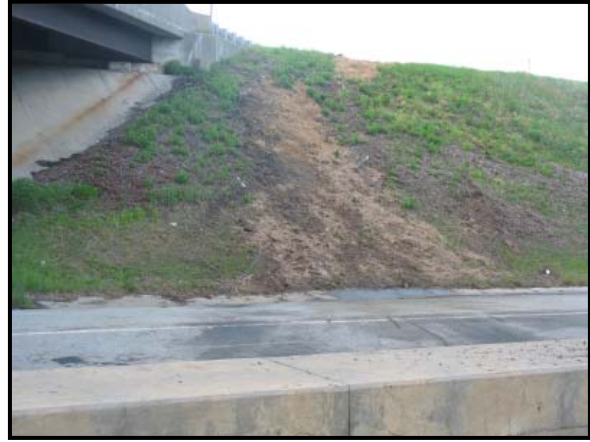
Figure 5: Look back view from final rest toward the embankment.
