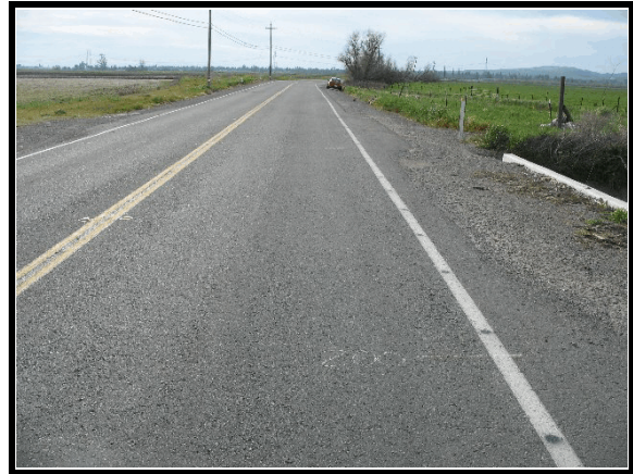
Figure 3. Approach to area of impact (west)
