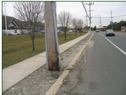
Figure 4. Struck utility pole.
