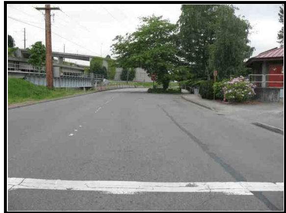
Figure 2. Southbound approach to impact with bridge rail
