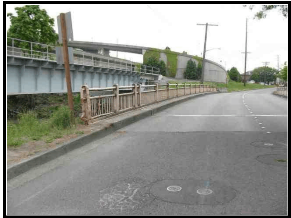
Figure 3. Impact with bridge rail
