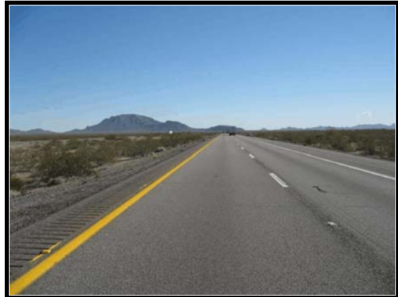
Figure 2. East approach to area of roadway departure
