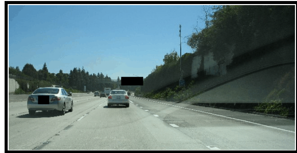
Figure 3. Southbound travel lanes
