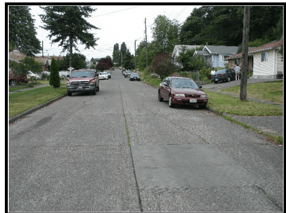
Figure 2. Approach to area of impact (north)
