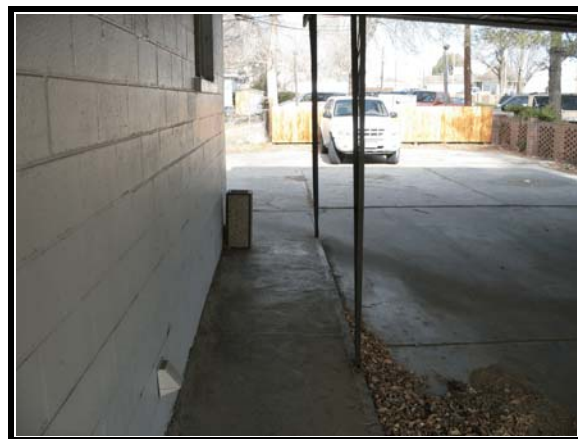
Figure 4. Path from door to parking area (north)
