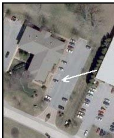
Figure 4: Overhead view of the incident site.
