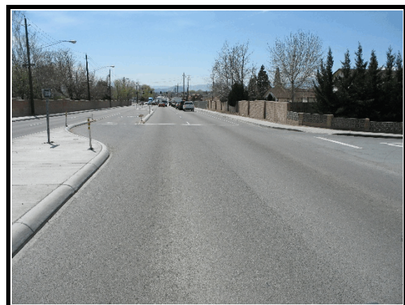
Figure 2. Approach to area of impact (south)
