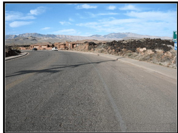
Figure 2. Approach to area of roadway departure (west)
