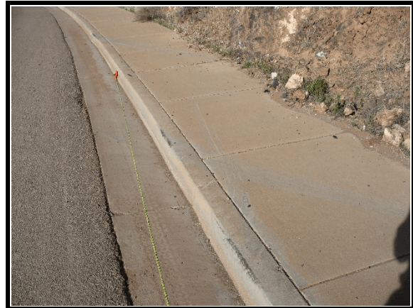
Figure 3. Area of roadway departure
