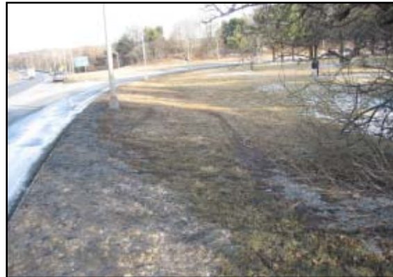
Figure 3. Left side tire marks on roadside.
