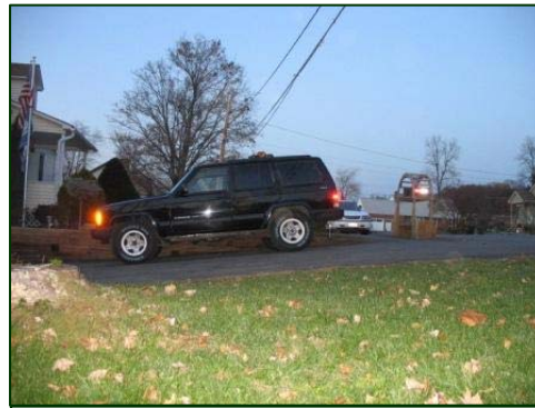
Figure 3. Lateral view of the driveway positive 13.5 percent slope.
