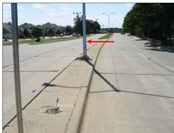
Figure 3: Arrow shows location of impacted luminaire pole, which has been replaced
