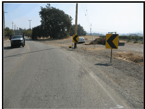
Figure 4. Area of roadway departure and impact with pole (pole has been replaced)
