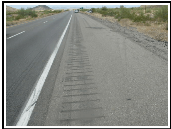
Figure 4. Vehicle path as it departs roadway toward trip point
