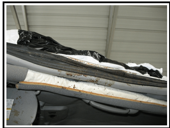
Figure 14. Left front roof rail contact
