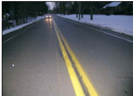
Figure 2. Overall view of the north/south roadway.
