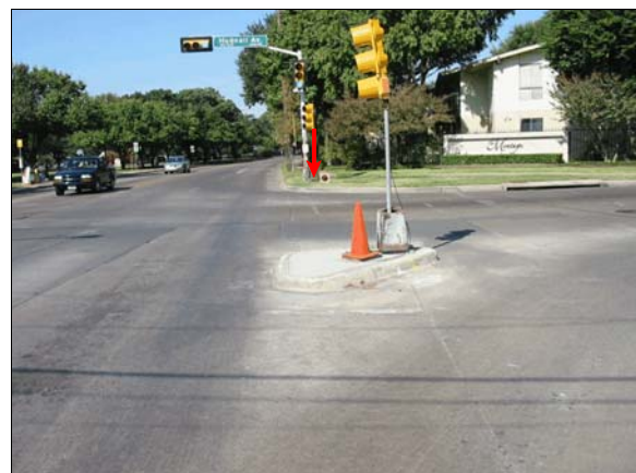
Figure 3: Overview of location of two struck traffic signal poles, pole in foreground was broken off its base, pole in background was displaced, arrow shows case vehicle's area of final rest
