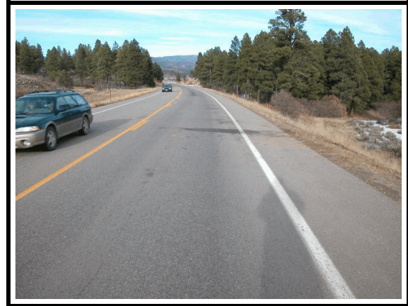
Figure 2. Area of impact—facing east
