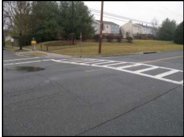
Figure 4: View of the northeast intersection quadrant.
