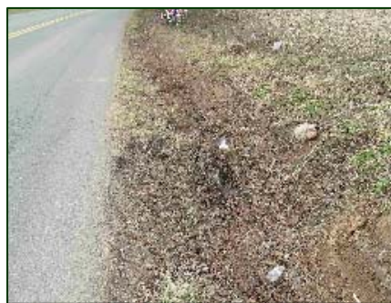
Figure 7. Culvert pipe and deepest point of the ditch.
