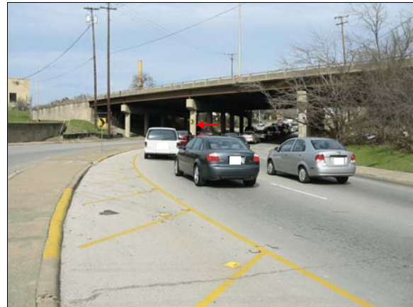
Figure 1: Case vehicle’s approach, northbound in outside lane, to impact with concrete bridge support (indicated by arrow)
