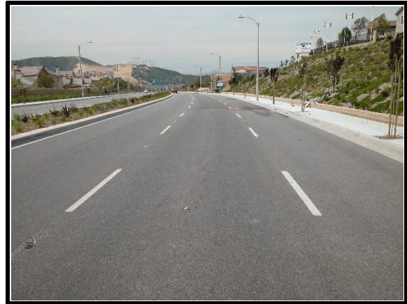
Figure 2. Approach to point of impact (west)
