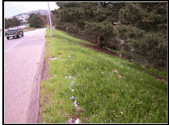
Figure 3. Area of road departure (North)
