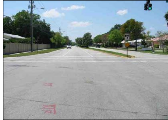
Figure 3 - Southbound view of the area of impact.
