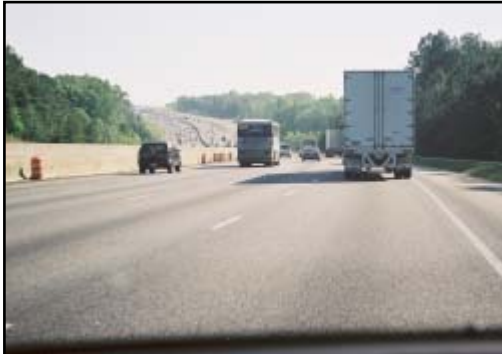
Figure 3. Approach from outboard travel lane
