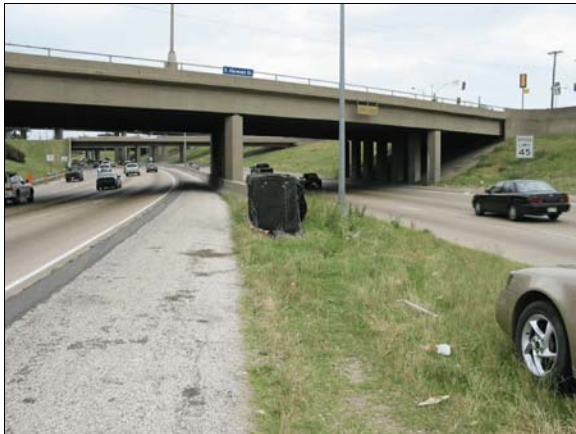
Figure 2: Approach of case vehicle to impact with the crash attenuator (case photo #04)
