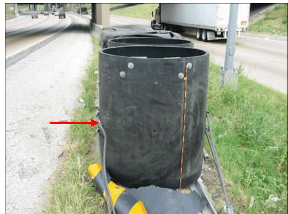
Figure 4: The crash attenuator impacted by the case vehicle, arrow shows plastic deposit from case vehicle's right headlamp, each stripe on rod is 5 cm (2 in) (case photo #06)
