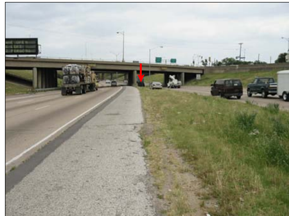
Figure 1: Overview of the trafficway and travel direction of the case vehicle to impact with the crash attenuator, indicated by arrow (case photo #01)
