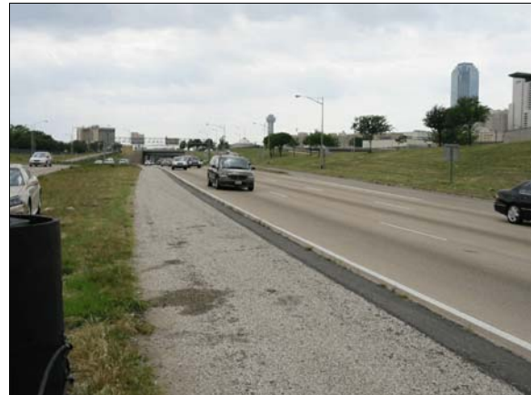
Figure 5: View west back to case vehicle's approach from the area of final rest (case photo #09)
