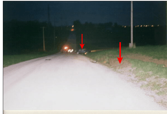
Figure 1: Police on-scene photo showing case vehicle's approach to roadway departure and final rest position; arrows show final rest and area of ditch impact and location where case vehicle became airborne (bare strip in grass to right of arrow in foreground is not crash related)
