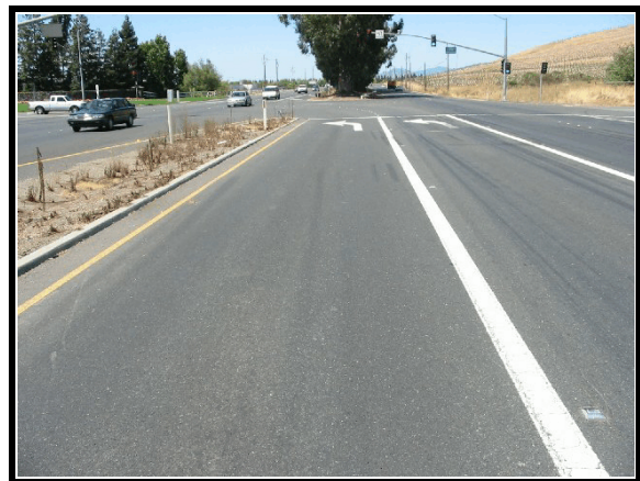
Figure 2. Approach to area of impact (north)
