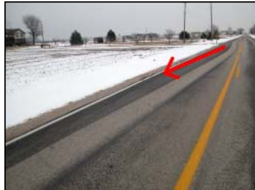
Figure 5. Area of trip-over and related roadway gouge
