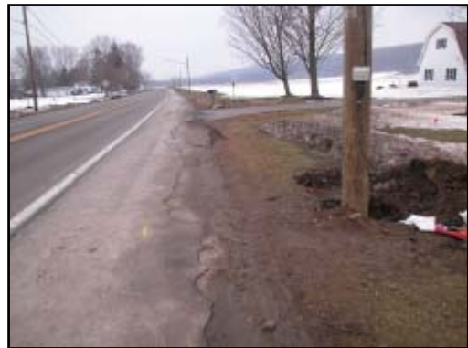
Figure 2. View of utility pole (replaced), driveway, and mailboxes (replaced)
