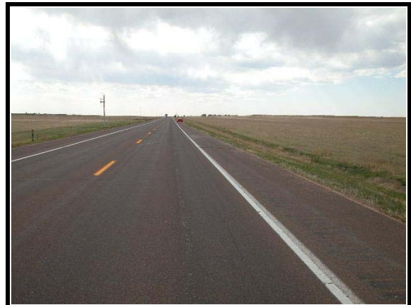
Figure 1. Approach to area of impact (east)
