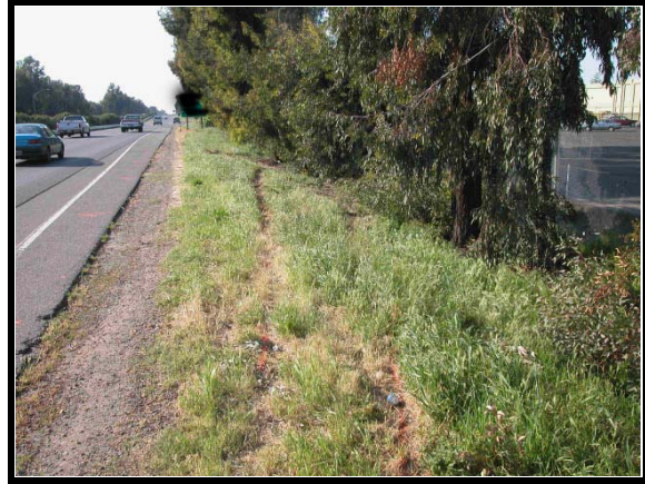
Figure 2. Approach to area of first and second tree impacts
