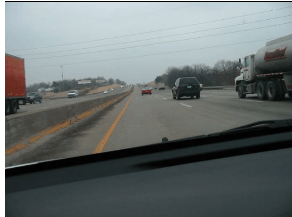
Figure 2: Approach of case vehicle northeastbound to impact with the concrete longitudinal median barrier (case photo #02)
