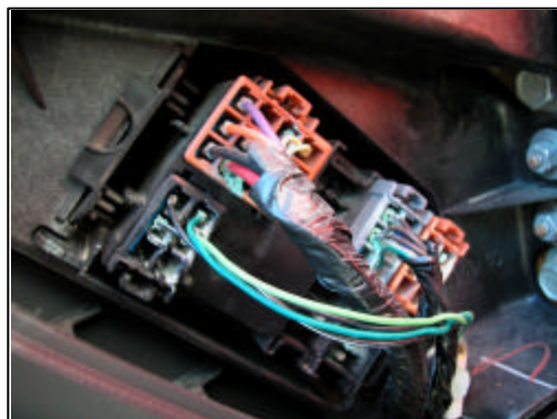
Figure 7. Right side fuse panel. Note oxidation from water damage.
