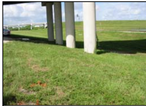
Figure 3. Impact to concrete overpass support.
