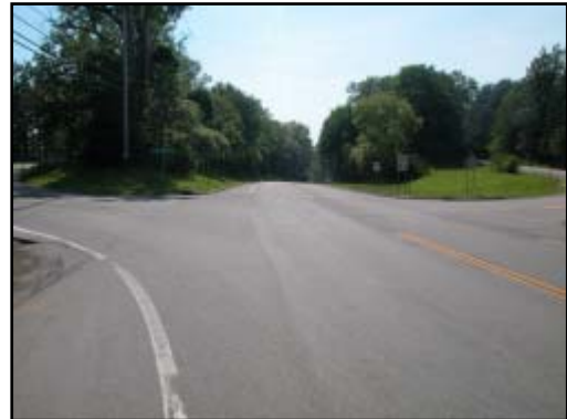
Figure 2. Northwest view of intersection.
