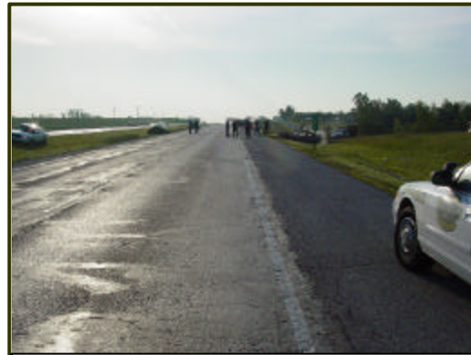
Figure 2. Overall eastbound view of the crash site on approach to impact.
