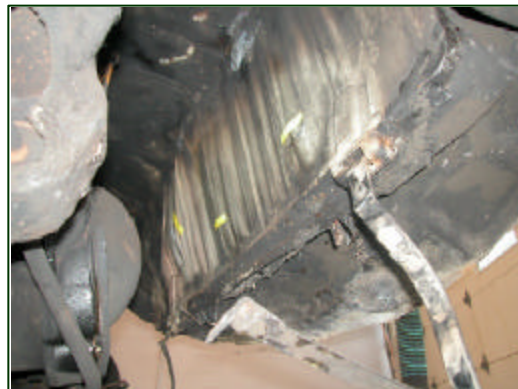
Figure 23. Outward dents on the forward wall of the trunk toward fuel tank from trunk contents .
