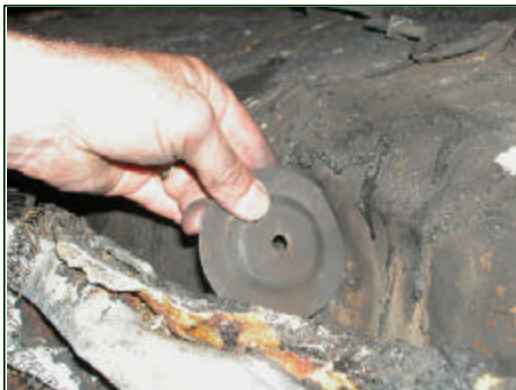
Figure 27. Penetration of the bracket washer through the trunk wall and into the back of the fuel tank.
