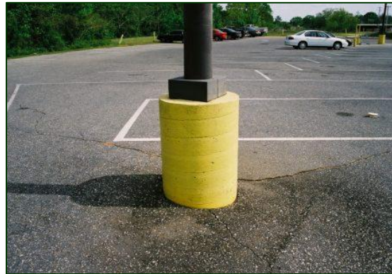
Figure 3. Struck pole base.
